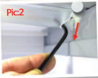
Next remove the diffuser/cover. This has a D shaped aperture at one end, usually the right-hand. Pull down using the diffuser Hook provided, this will free the diffuser from its front and rear grooves as in **Pic:2**.
